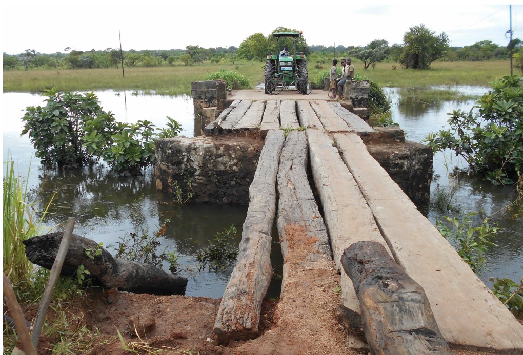
Maintenance of infrastructures in a Hunting Area, Mozambique (©Jean-Baptiste Deffontaines/IGF Foundation)
