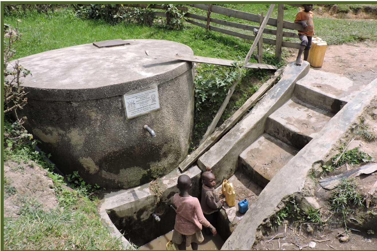
Plate 2: Protected spring with reservoir tank at Kitahurira Parish, Ikumba S/C, Rubanda District
