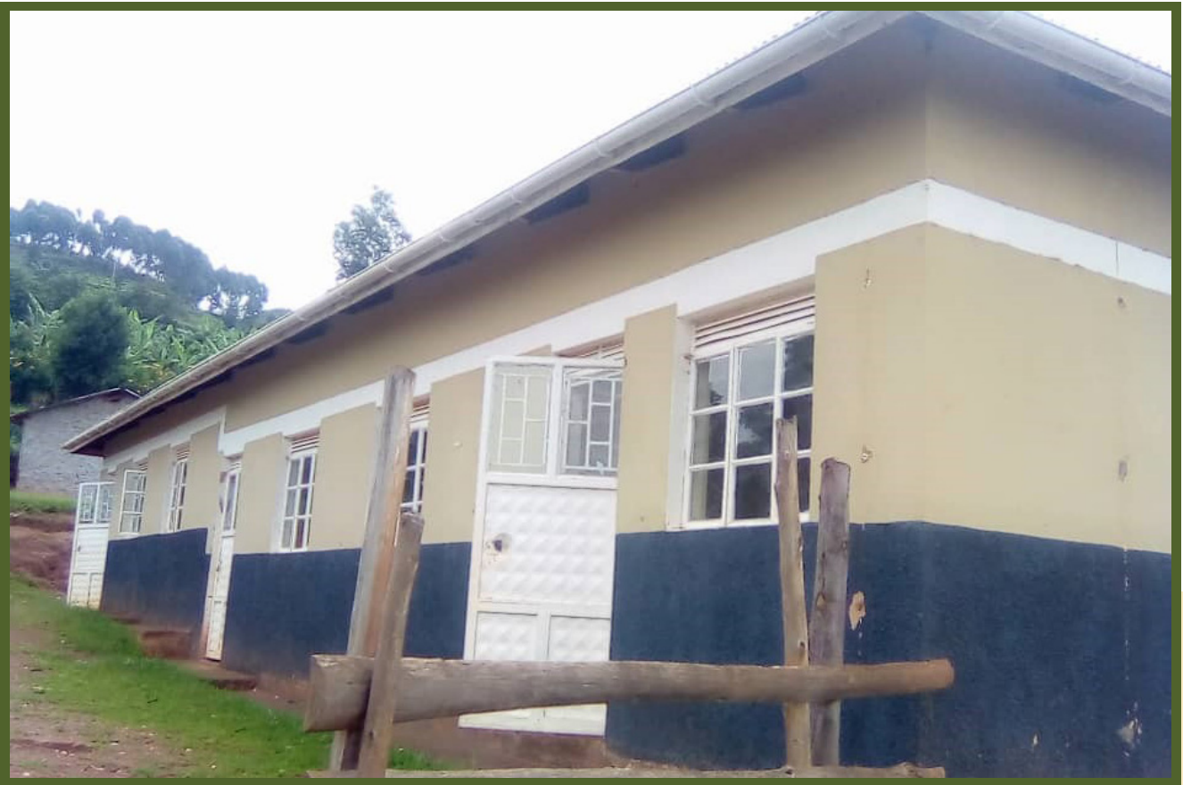
Plate 4: Two classrooms block and office at Kyogo Annex Primary School, Kashekyera Ward, Ruhija Town Council, Rubanda District
