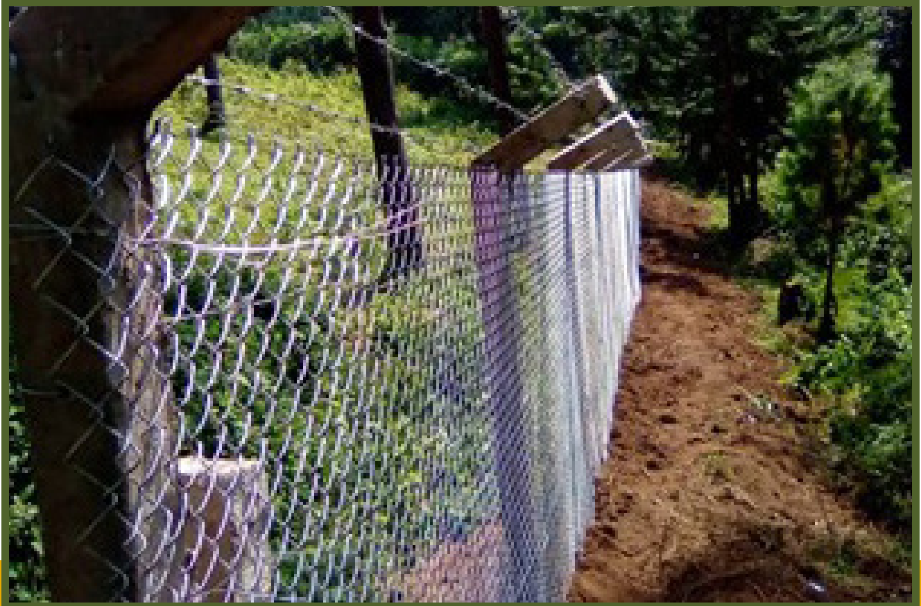
Plate 6: Chain link constructed at Mataka and Kyeitokwa villages in Ntungamo and Kiyebe parishes in Ruhija S/County Rubanda District.
